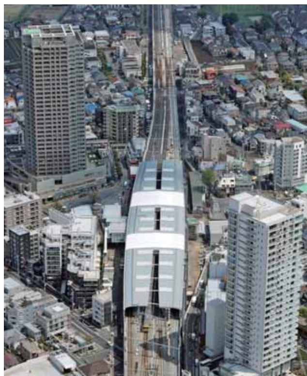
Japan Railway Construction, Transport and Technology Agency (JRRT)/ Railway Construction Projects Private Rail Line “Quadruple track construction by high bridges”/ Seibu Ikebukuro Line, Tokyo (Nerima - Shakuji Ko-en (4.1km))
