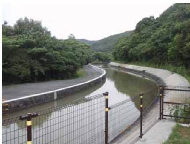
Japan Water Agency/Toyogawa Canal System Reconstruction and Management Department/ Futagawa Open Canal/Toyohashi City, Aichi Prefecture
