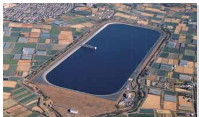
Japan Water Agency/Toyogawa Canal System Reconstruction and Management Department/ Bamba Regulating Reservoir/Toyohashi City, Aichi Prefecture
