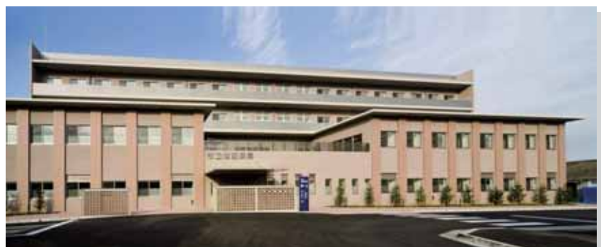
Local government/Hospital Project/ Bizen Municipal Hospital/Bizen City, Okayama Prefecture
